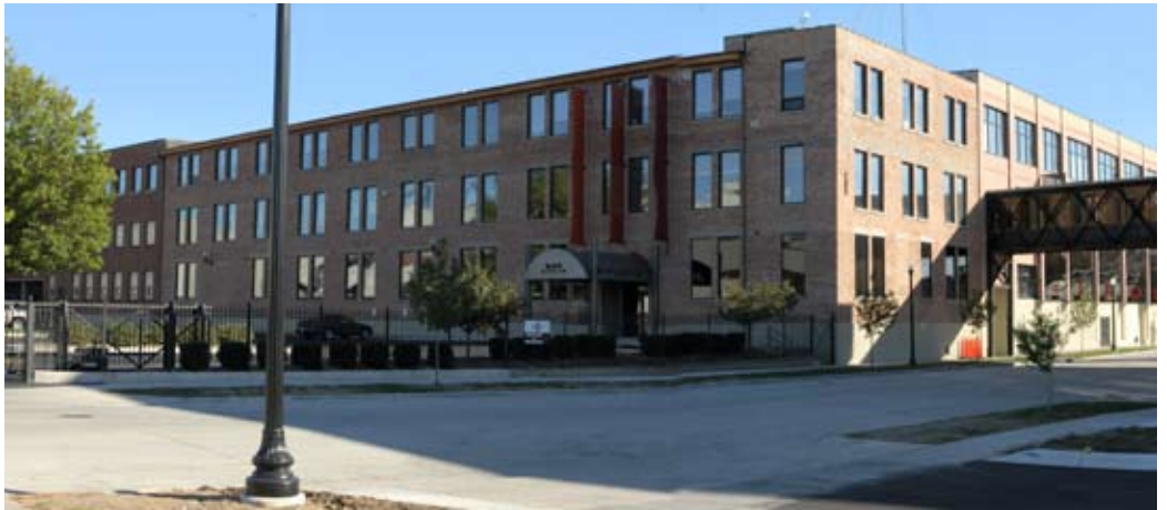
Hendricks Commercial Properties purchased the site of a former machinery plant and transformed it into Beloit Ironworks. Hendricks' headquarters are now located in the complex.
